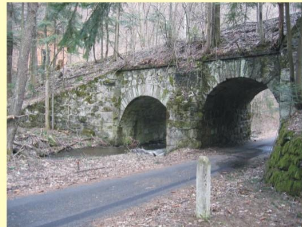
Stav 2005 Bridge in 2005
