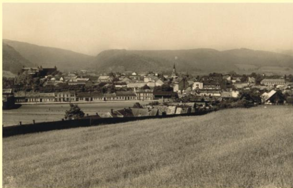
Zvolen, priestor za malou železničnou stanicou pred výstavbou budovy, koniec 20. rokov 20. storočia Zvolen, the site behind the town railway station prior to the building construction (1920s)
